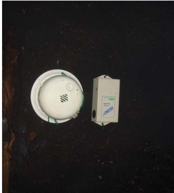
UCB Particulate Matter Monitor and HOBO CO Logger
